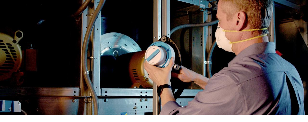
With this test, the air mixing ratio was set to 20% outdoor air and 80% return air. We installed a total of eight Opti-Lok devices according to the system size, with one unit per 3,800 CFM per air source. Two units were applied to outdoor air, and six units were applied to the return air. In this particular case, the team did not have access to apply the return air units in the most ideal location.
